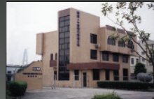
Factory Fujian, China
